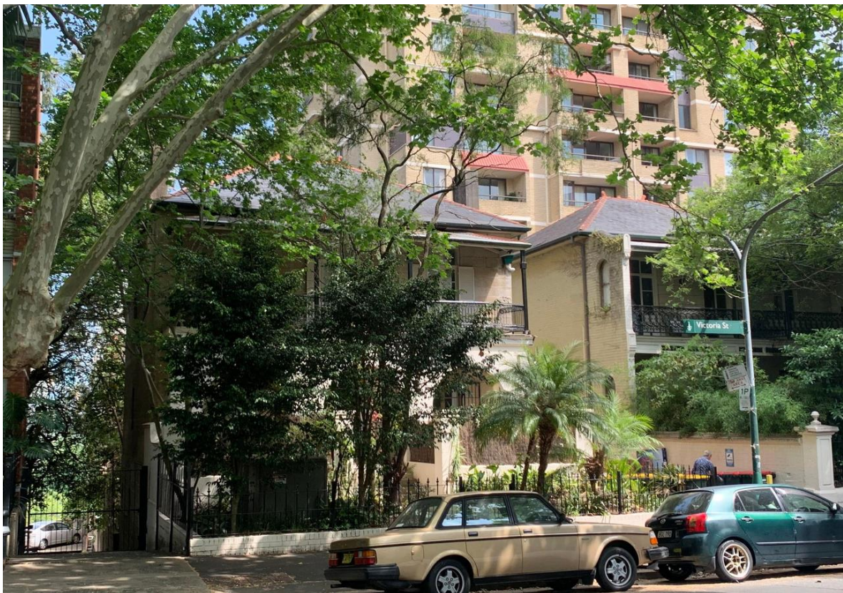
Figure 4: Adjoining heritage items to the northeast at 101-115 Victoria Street, viewed from Victoria Street
