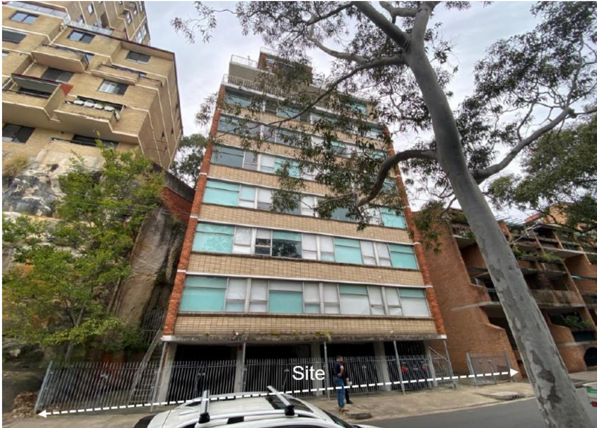
Figure 3: Site viewed from Brougham Street, looking east
