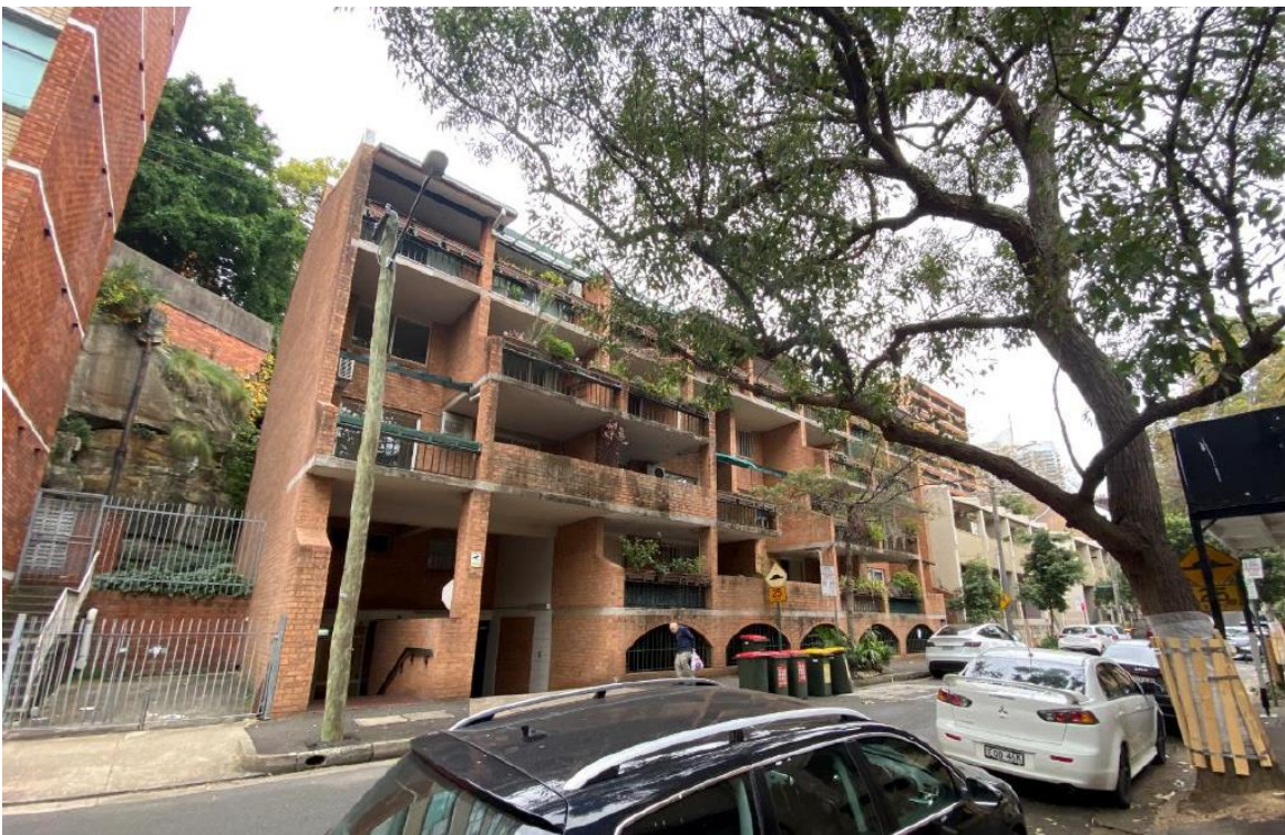
Figure 6: Adjoining buildings to the southwest at 30A-34 Brougham Street viewed from Brougham Street
