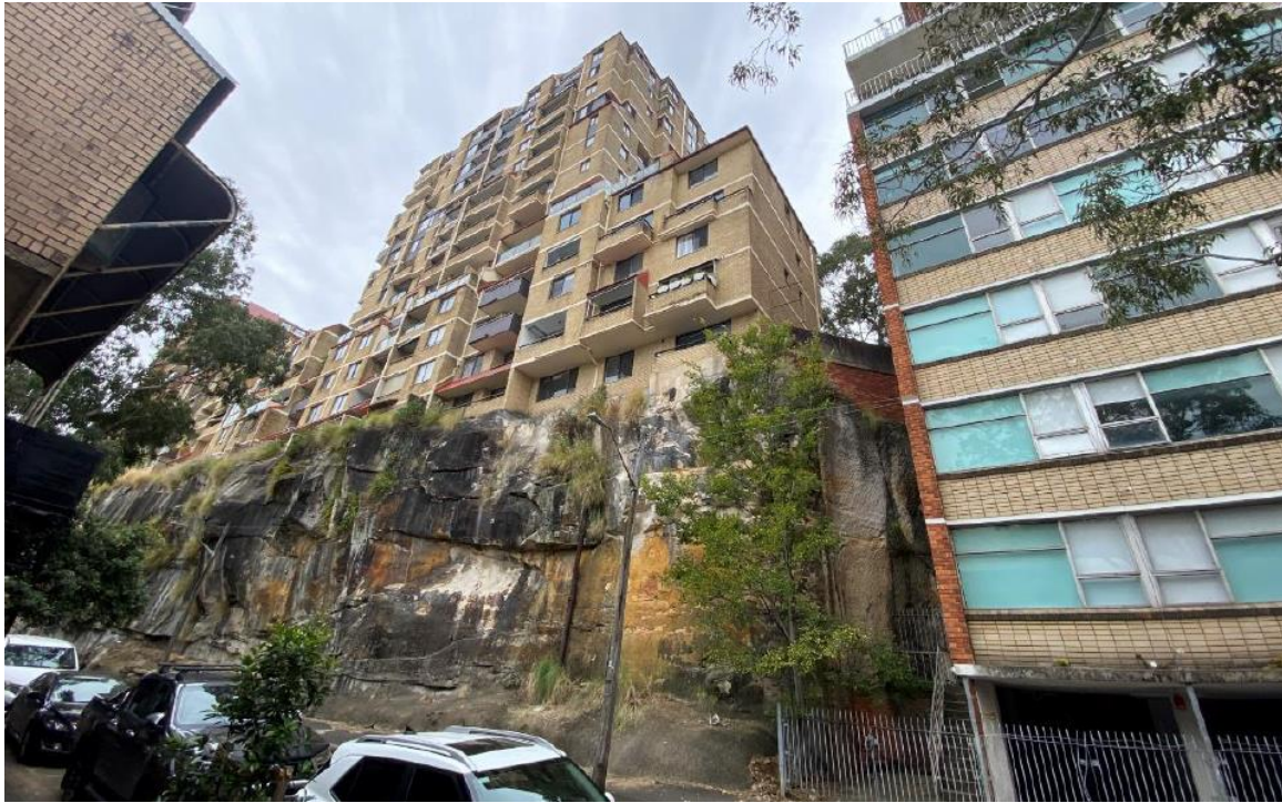
Figure 7: Adjoining buildings to the northwest at 101-115 Victoria Street, viewed from Brougham Street
