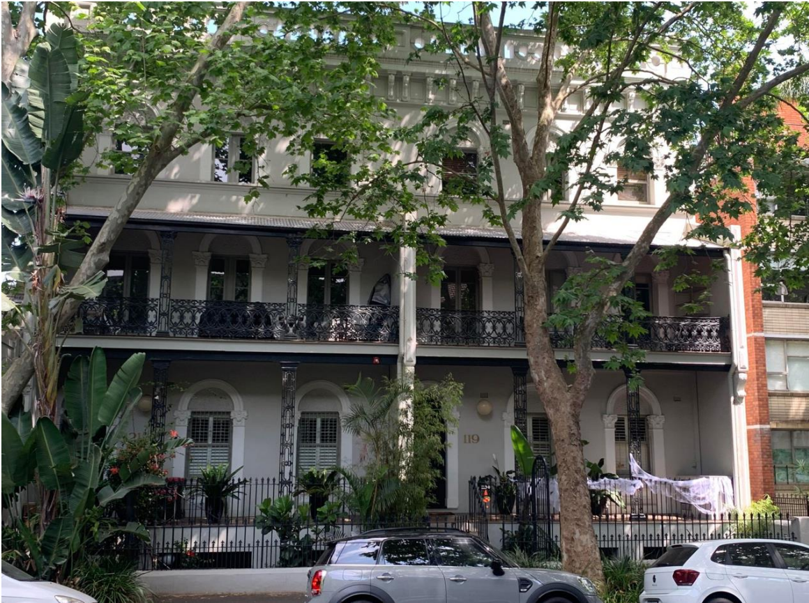
Figure 5: Adjoining heritage items to the southeast at 119-121 Victoria Street, viewed from Victoria Street
